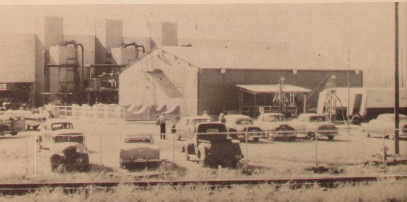
Liquid oxygen plant, Aerojet-General Corporation, Azusa, California
